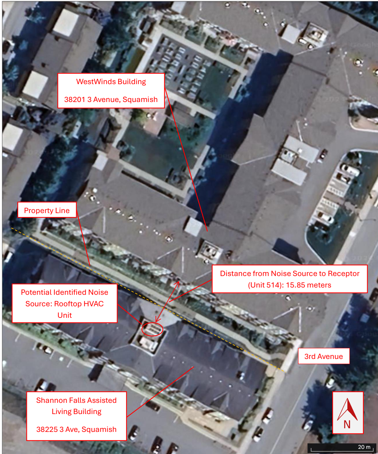
Figure 1 - Aerial view of shared southern property line between WestWinds (38201 3 Avenue, Squamish) and Shannon Falls (38225 3 Avenue, Squamish) residential buildings and distance from potential identified noise source and receptor (Image: Google Earth – Accessed September 3, 2024).
